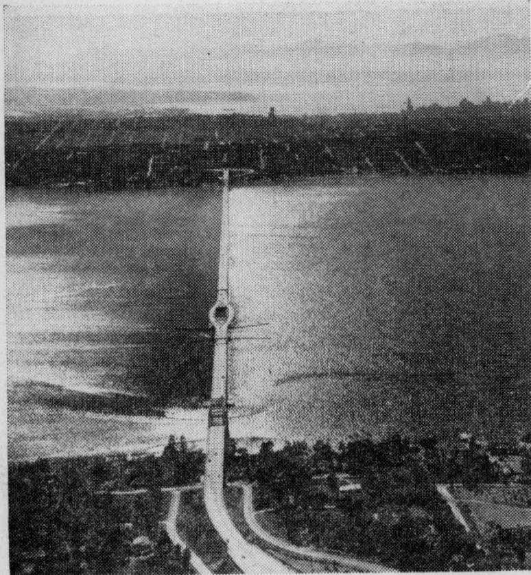
LAKE WASHINGTON'S floating bridge, the longest in the world can be seen connecting Mercer Island to the city of Seattle. Elliott Bay and the Olympic Mountains are in the background.
