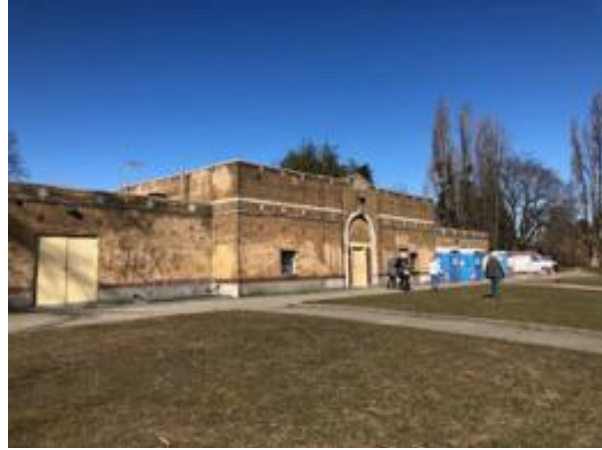
Green Lake Bathhouse, east façade. Photo by Cristin Miller.
