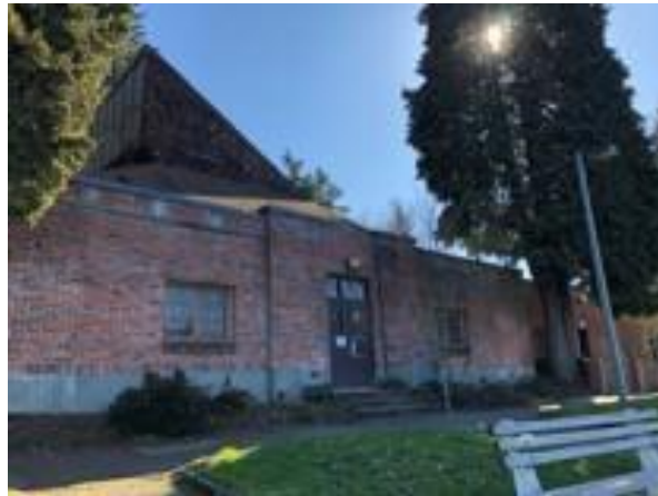
Seward Park Bathhouse, south façade. Photo by Cristin Miller.
